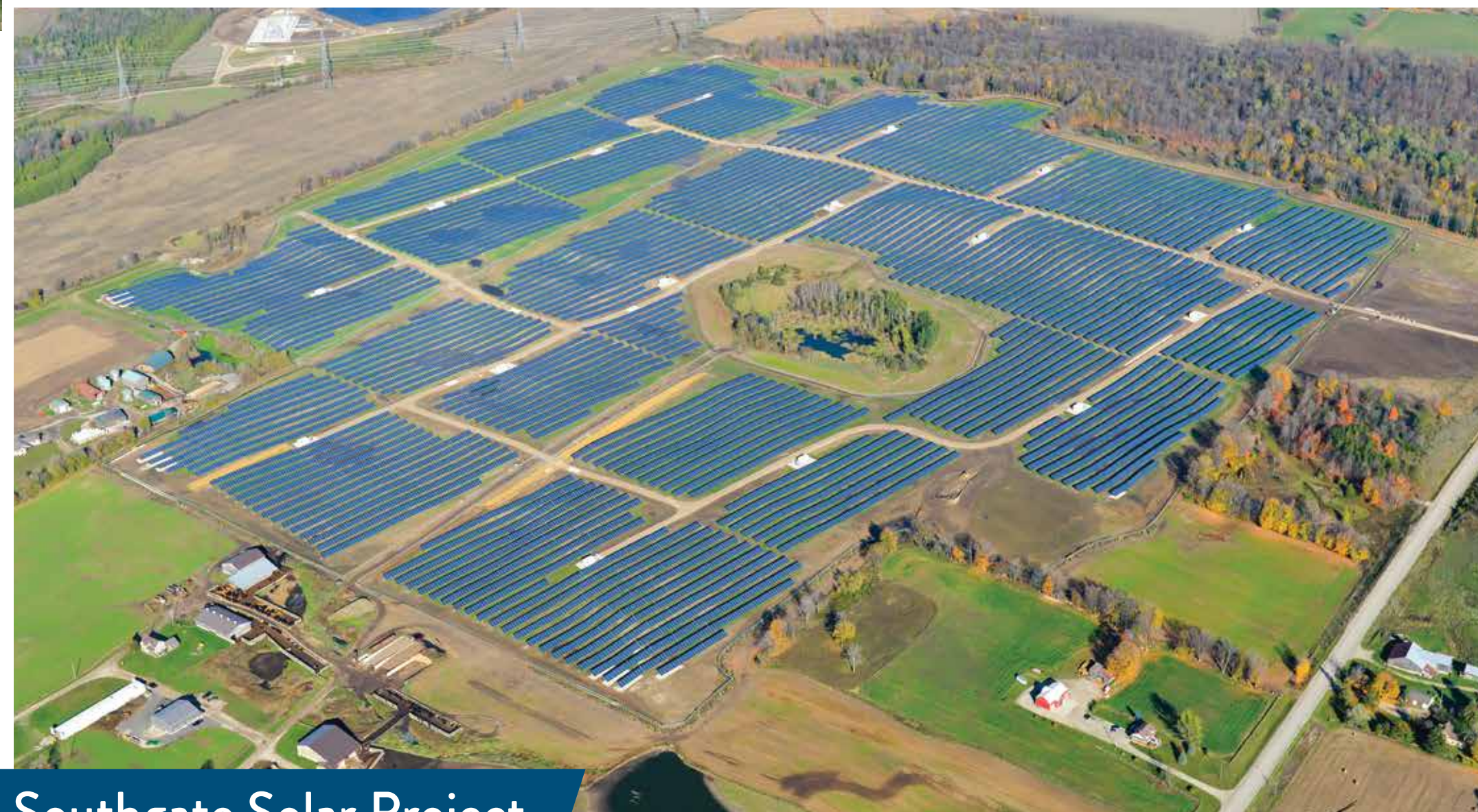
Southgate Solar Project
